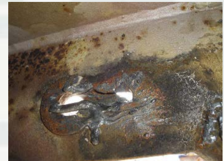
Flame cut drain holes
