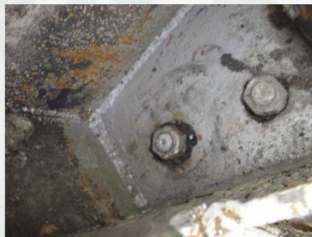
Corrosion around socket bolts
