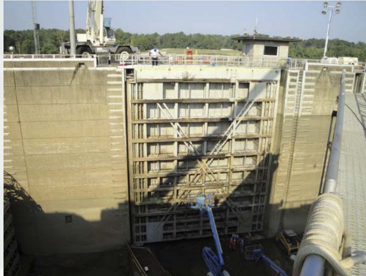
Corrosion at Claiborne Lock due to inadequate CPC systems
