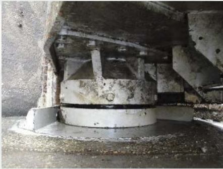
Pintle socket during dewatering
