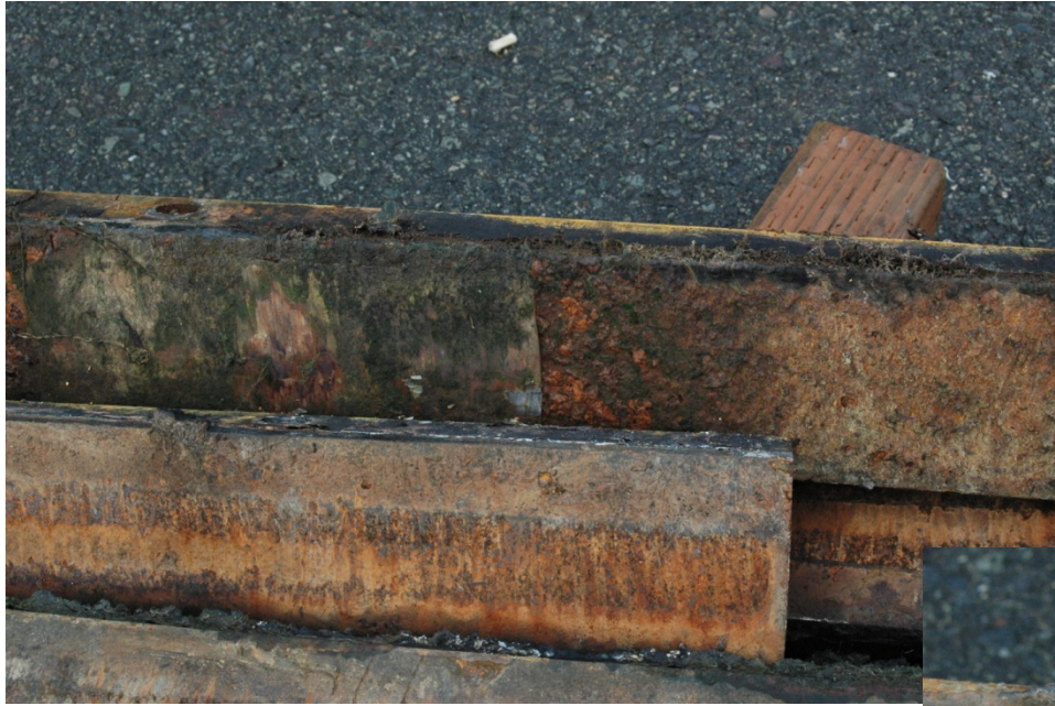
Very corroded existing steel blocks.
