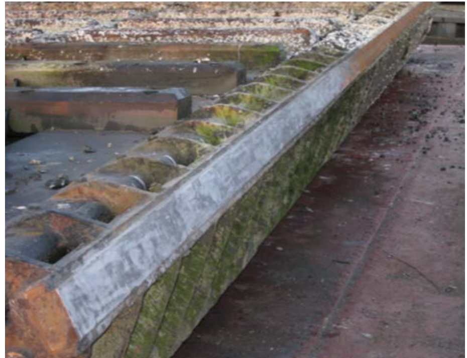
Corroded steel miter blocks.
